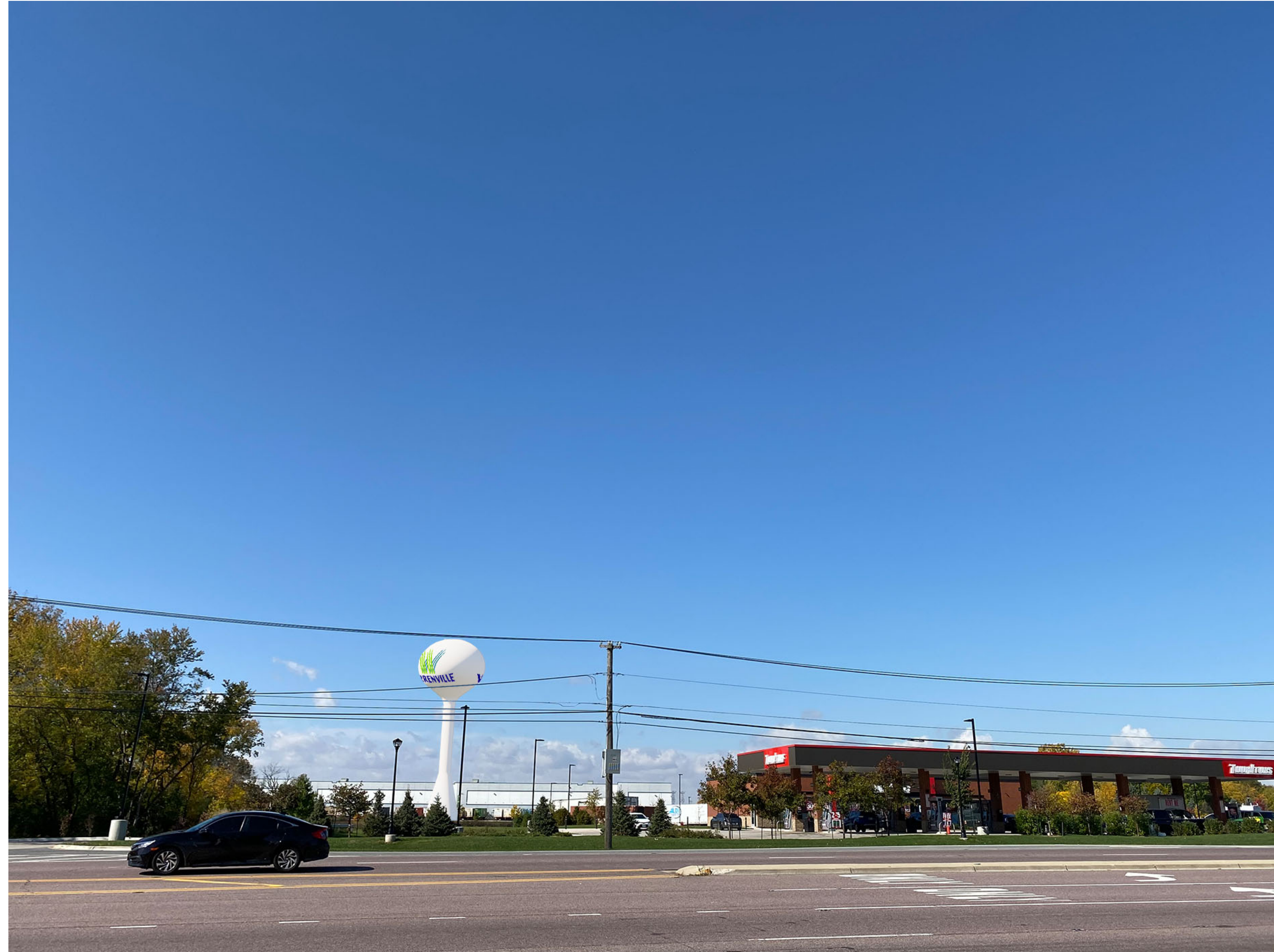
WATER TOWER FROM ACROSS RT 59
