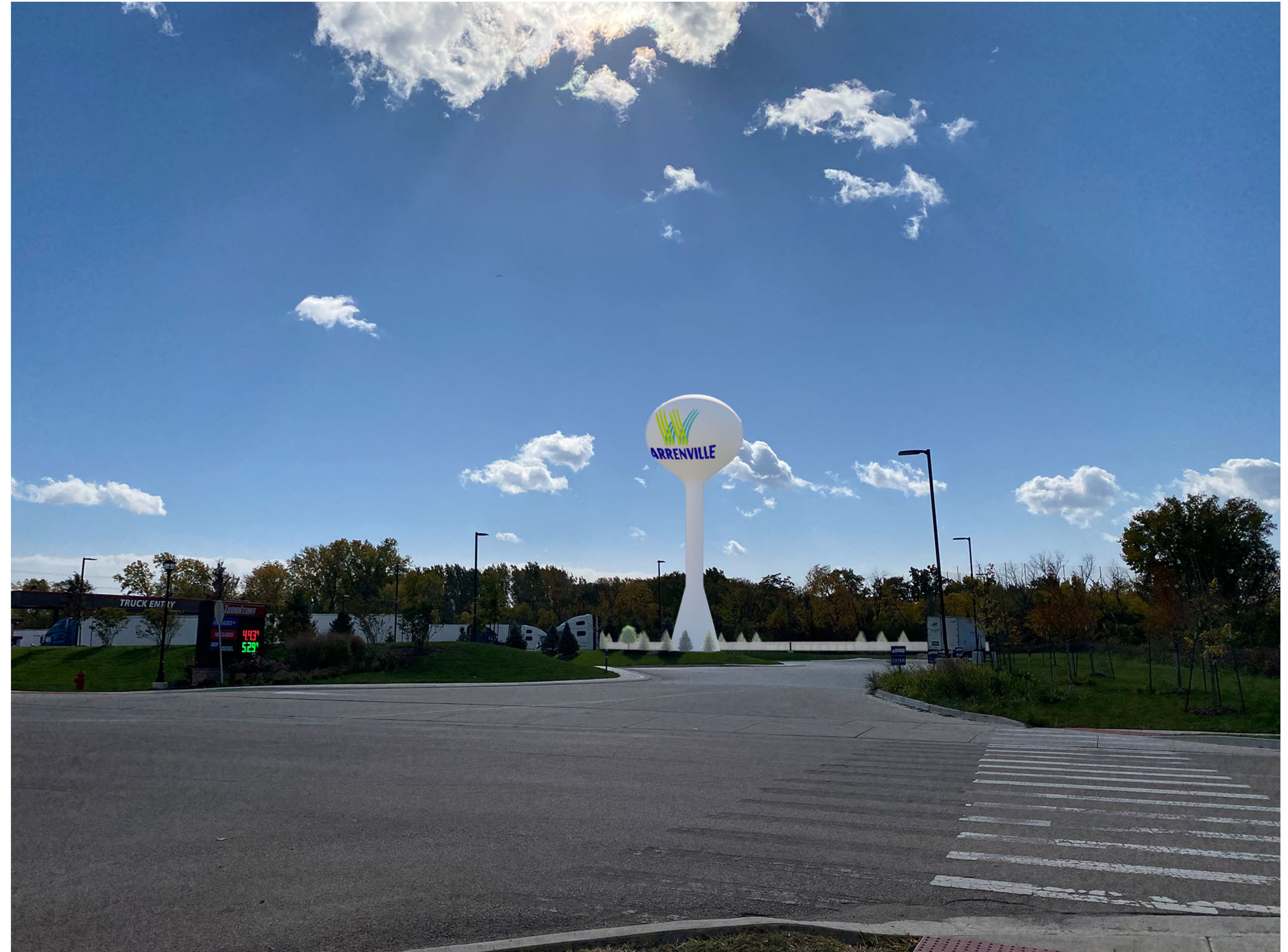
WATER TOWER FROM CORNER OF DUKE & BARKLEY
