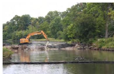
Warrenville Grove Dam Modification
